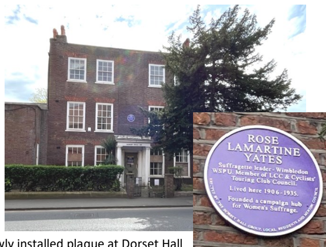
Newly installed plaque at Dorset Hall
